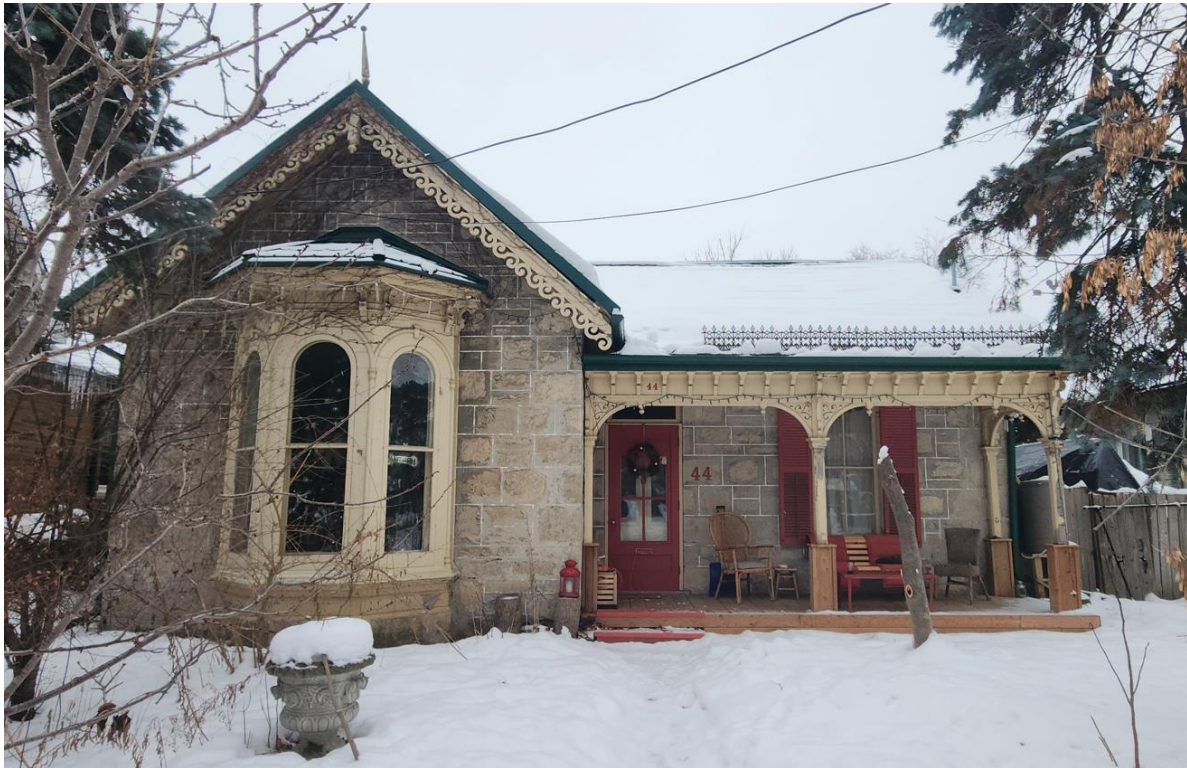
Figure 2 – 44 Edinburgh Road North from street. (Heritage Planning 2025)
