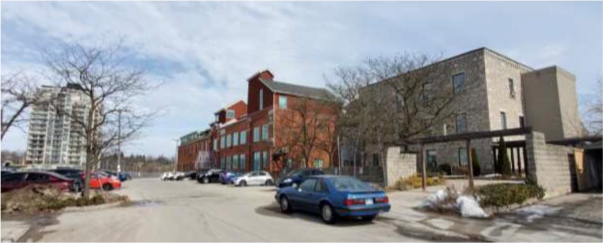
Figure 12 - 111 and 97 Farquhar Street.
