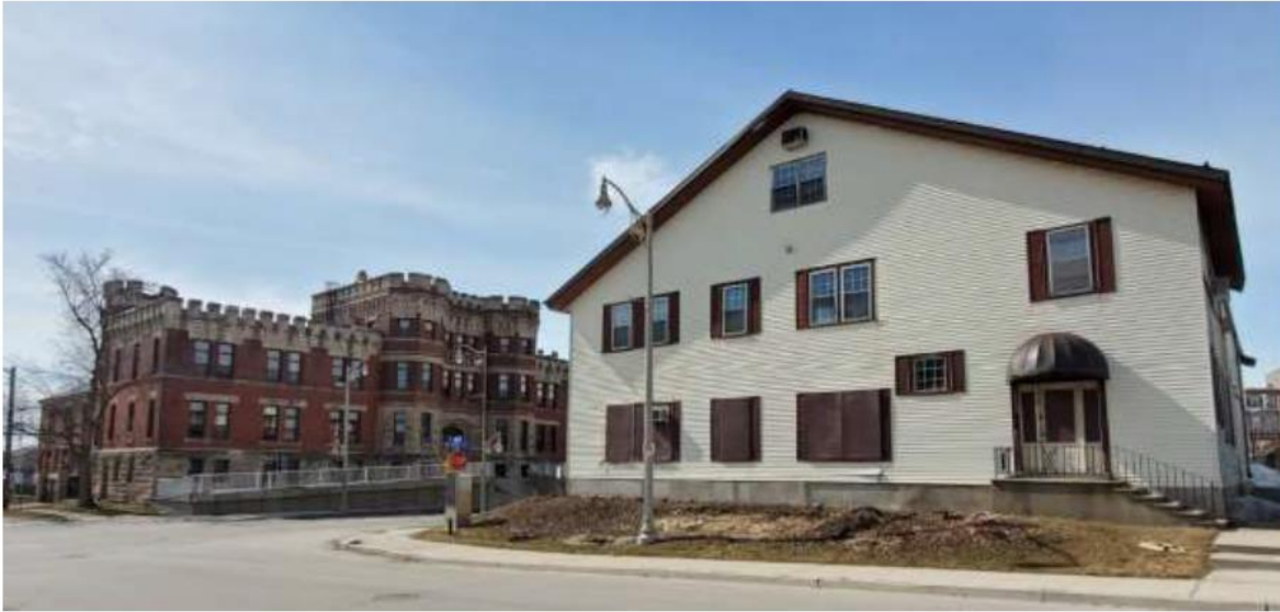
Figure 15 - Armoury at 7 Wyndham Street North and Drill Hall at 72 Farquhar Street.
