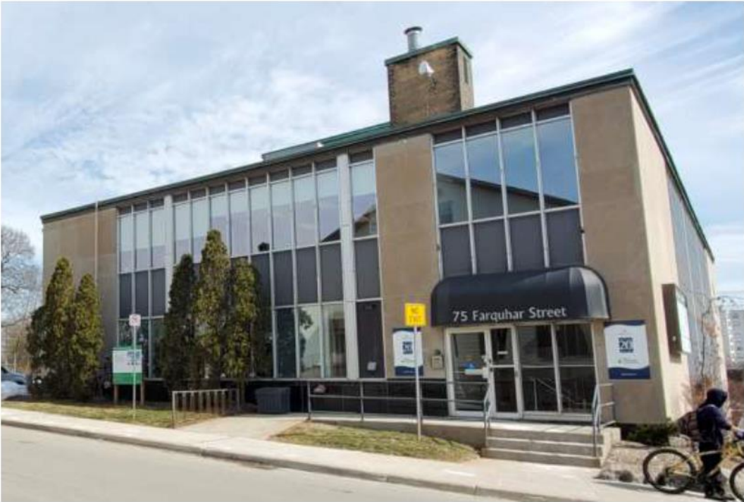
Figure 1 – Subject building fronting Farquhar Street.
