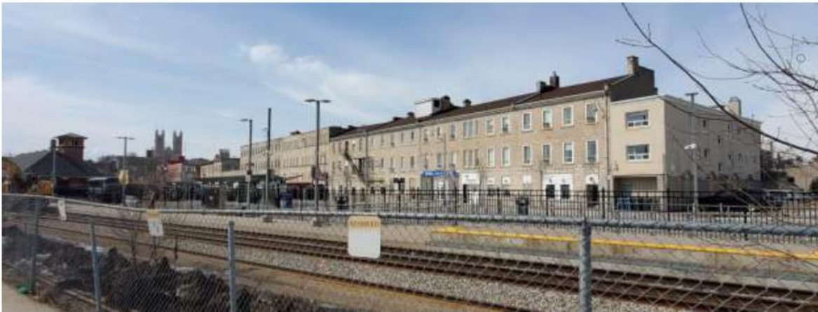
Figure 16 - Carden Street from Farquhar Street.
