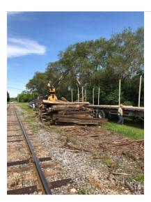
**Ballasting and surfacing program:** New track ballast was delivered and distributed to MP 16.35 –25.84. Track surfacing brings the level of the track to new standards of safety, providing maximum performance and extending the life cycle of track components. Ballasting provides a stable base for the track and allows for better drainage which extends the life of the ties.
