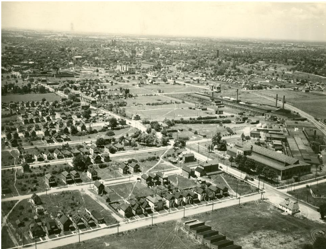
Figure 2: View of York Road at Victoria Road, 1948 (Guelph museum)
