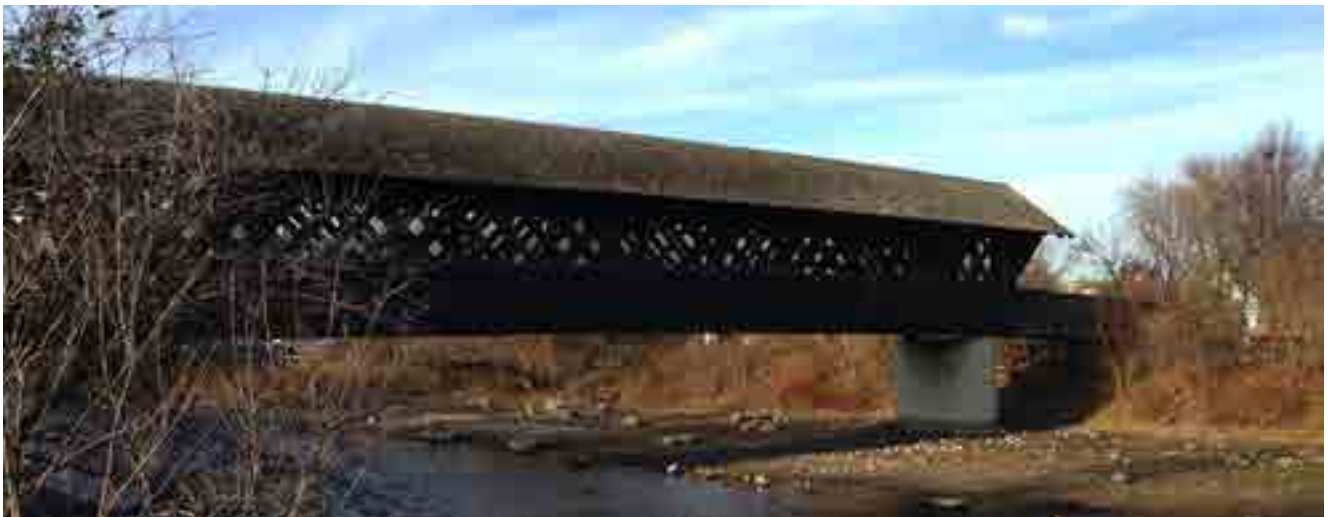
Figure 1.4.1. Timber Pedestrian Bridge in Guelph, Ontario (Photo Credit: E. Chau)
