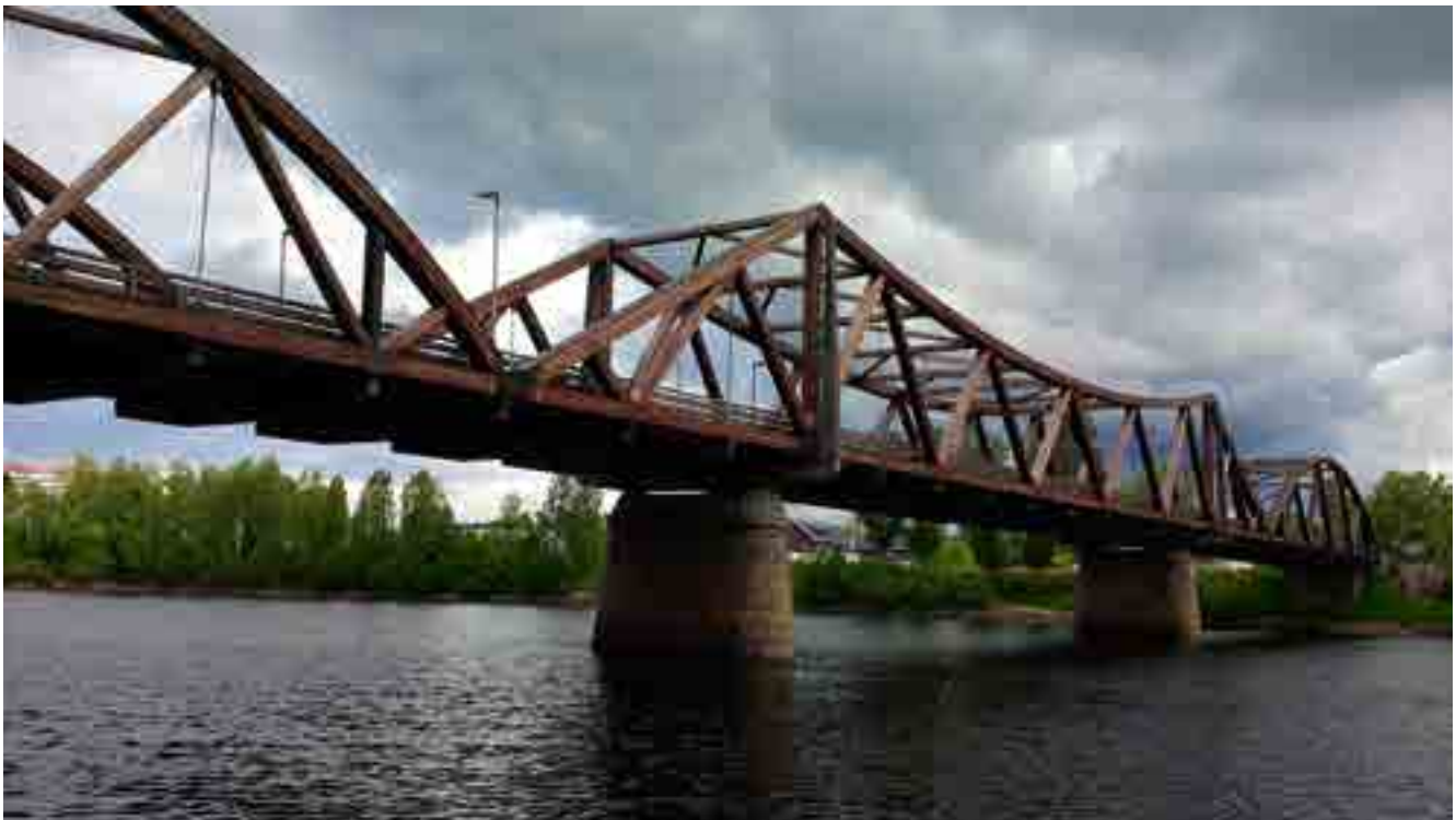
Norwegian Bridge with member protection. Photo Credit: FPIinnovations
