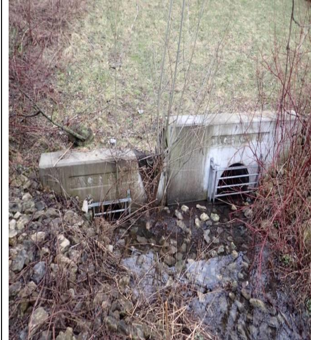
Photo C: Upstream section - right bank culvert
