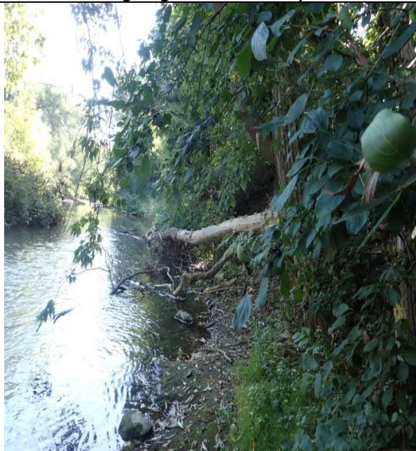
Photo I: Downstream section - left bank looking downstream, large woody debris and overhanging vegetation cover
