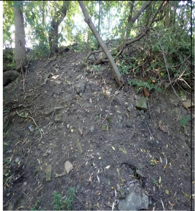
Photo H: Downstream section - left bank erosion
